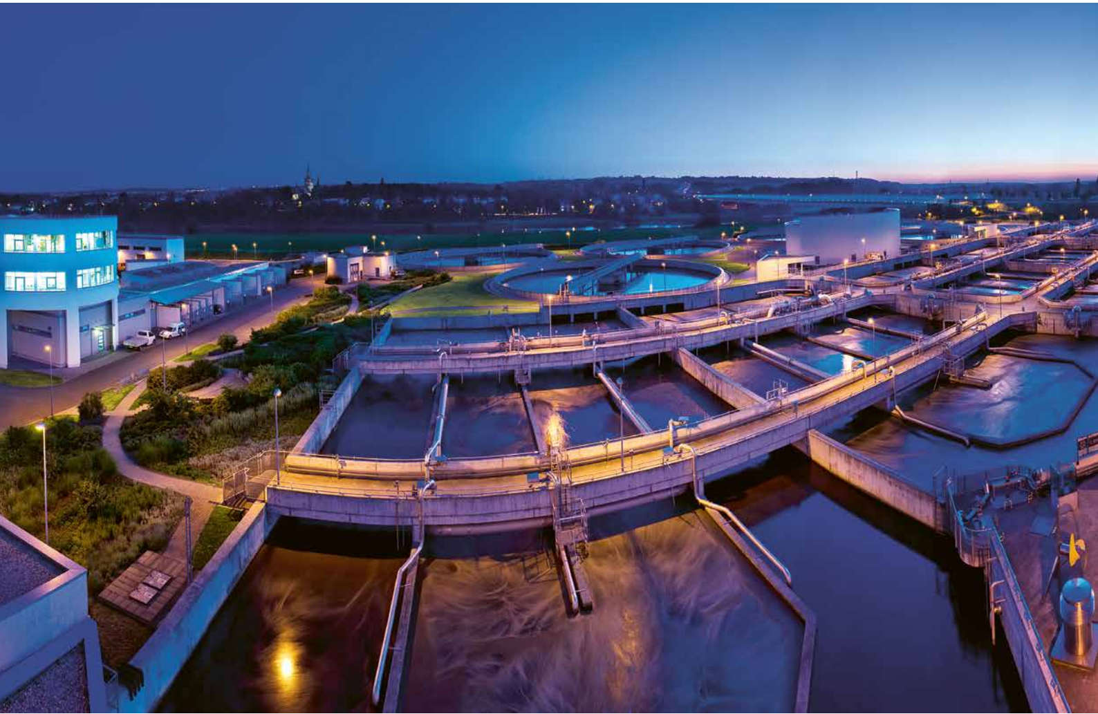
▲ Water treatment plant in Dresden.
