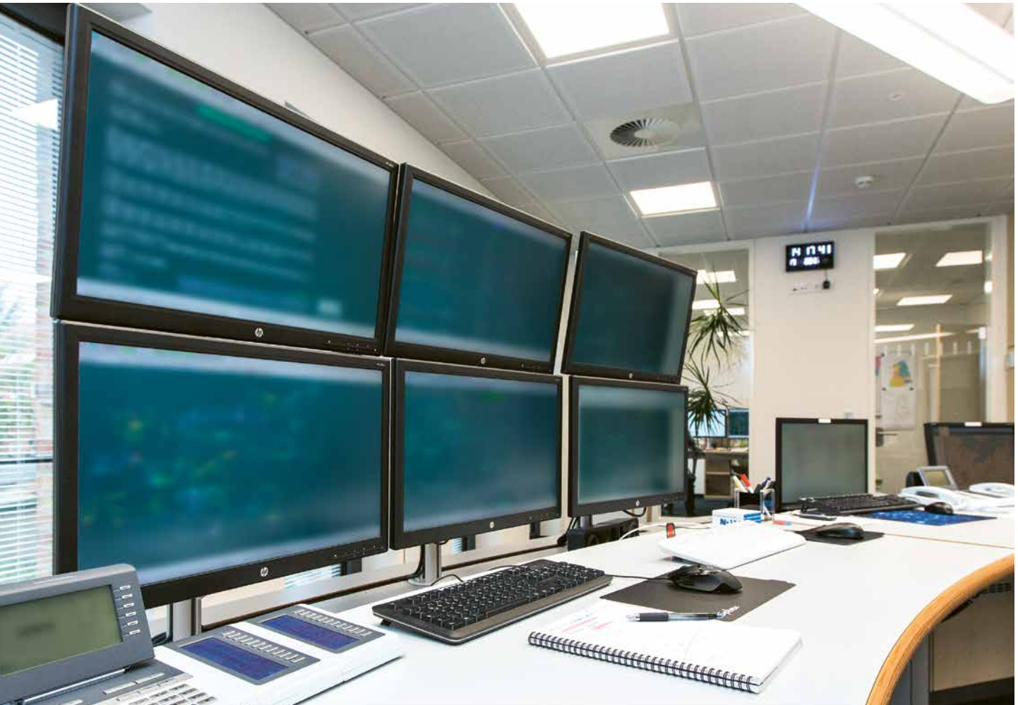
▲ View of the WEMAG Netz GmbH grid control centre, where the Intelligent Reactive Power Management System (IRPMS) is deployed.
